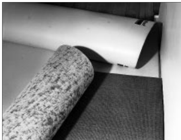
3) Glue down the widths at right angles with the padding
