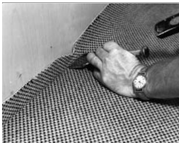
8) Knock down the carpet into the angle between floor and wall
