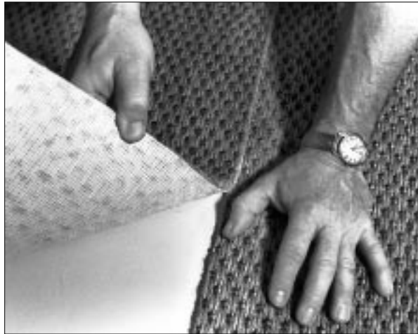
5) The next widths should overlap by 1 - 2 threads
